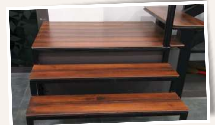
Flooring used in stair case
